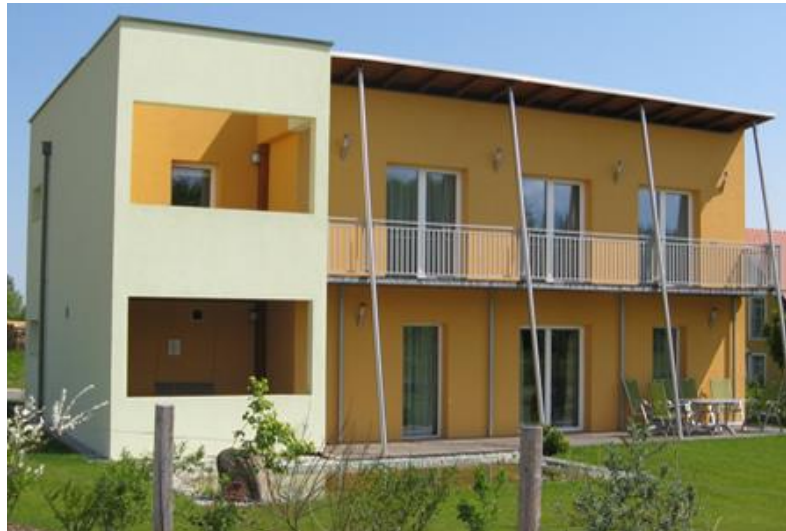
Figure 3: Example passive house in Großschönau
